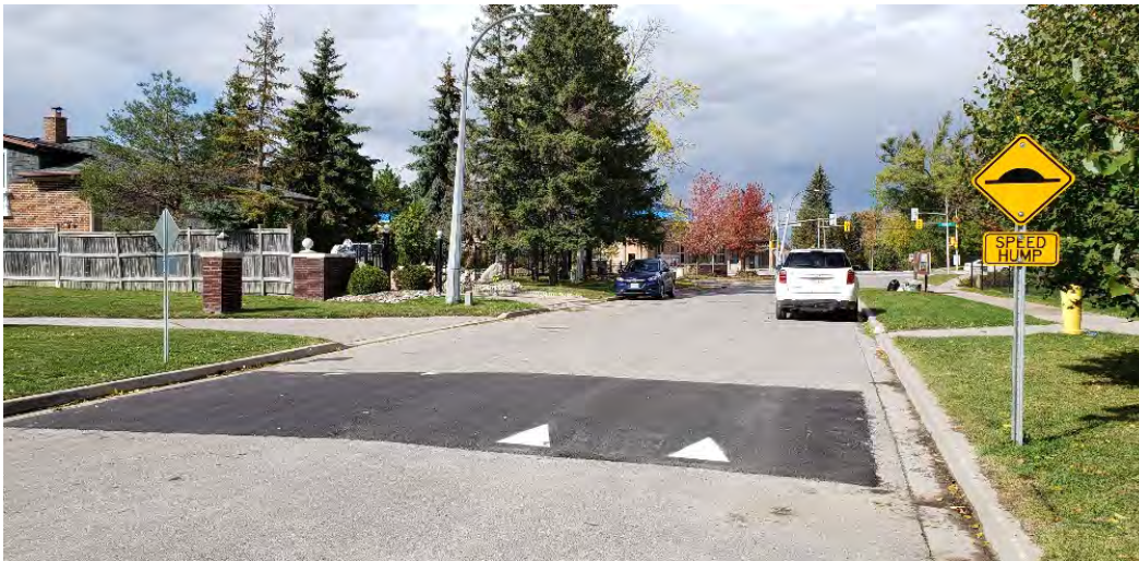
Figure 3-3 Speed Hump Installation Example on Banner Lane
