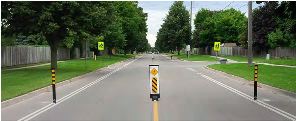
Figure 3-1: Typical Flexible Bollard Installation
