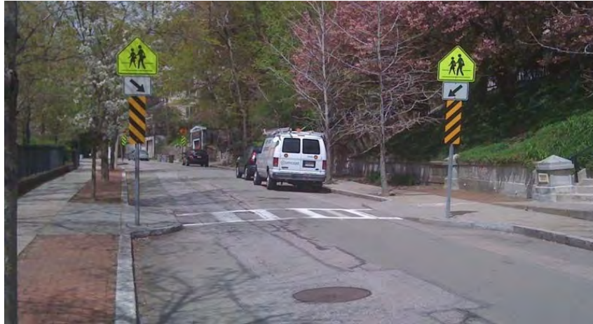
Figure 3-4 Curb Extension Example
