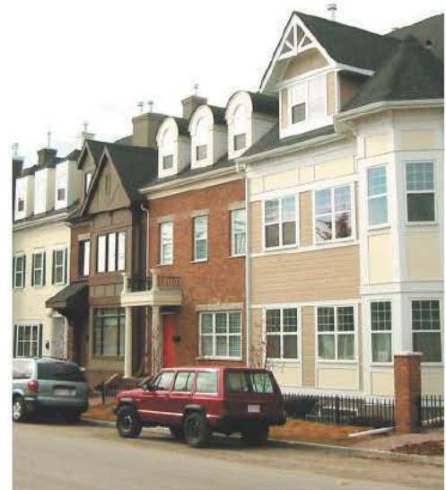
Figure 4.16 A variety of façades contribute to a common setback.
