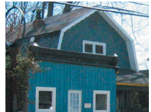
Figure 4.19 A variety of roof styles and building materials are found in Schomberg.
