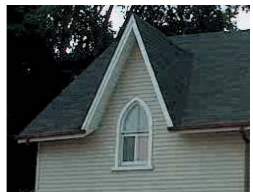
Figure 4.20 Peak roofs are recommended to mitigate additional building heights above the existing two storey urban fabric
