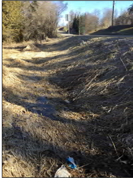
Photo 1: HDF A, facing north (April 3, 2020)
