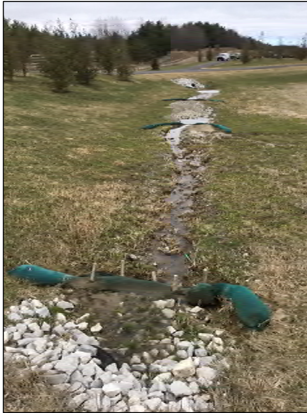
Photo 8: Western portion of HDF H, facing west (April 3, 2020)
