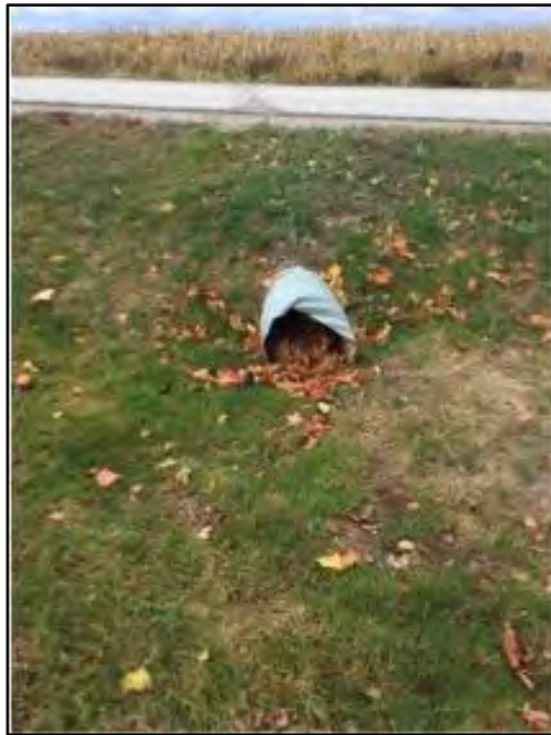
Photo 3. Upstream view from south side 15 th Sideroad (November 3, 2016)
