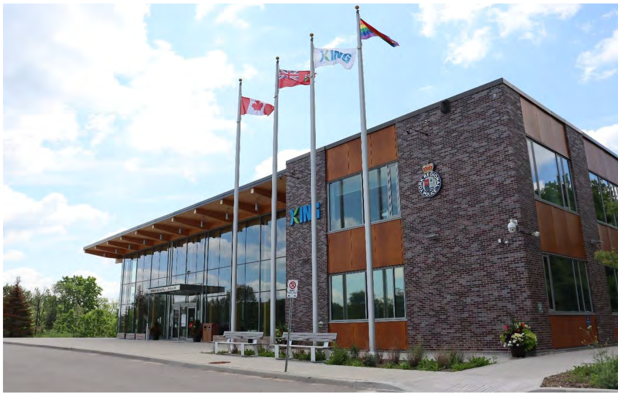
King Township Municipal Centre (KTMC)
