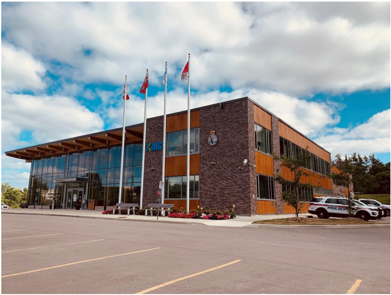
King Township Municipal Centre (KTMC)
