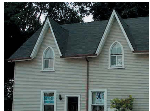
Figure 4.22 Peak roofs are recommended to mitigate additional building heights above the existing 2-3 storey urban fabric
