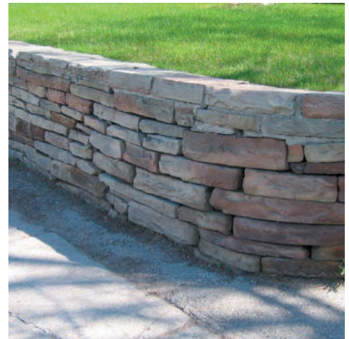
Figure 4.29 The existing stone wall on King Road is a wonderful means of transitions heights. A more durable natural stone retaining wall product should be used to maintain the look and feel of the original wall in the event it needs to be replaced.
