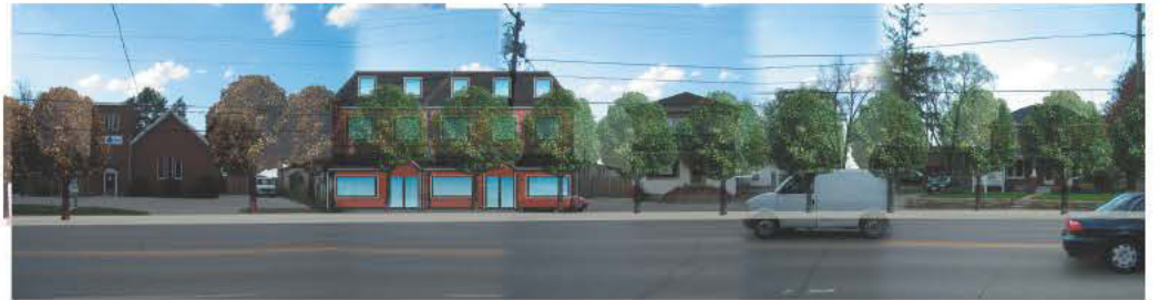
FIGURE 6.12 - NORTH SIDE OF KING ROAD CONTINUING FROM ABOVE
