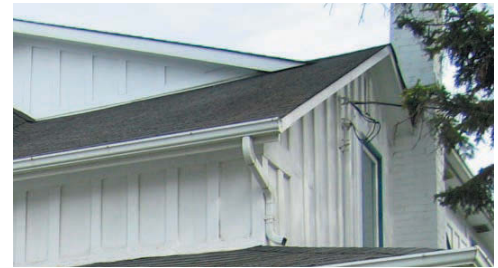
Figure 4.21 Many different roof styles are found in the area
