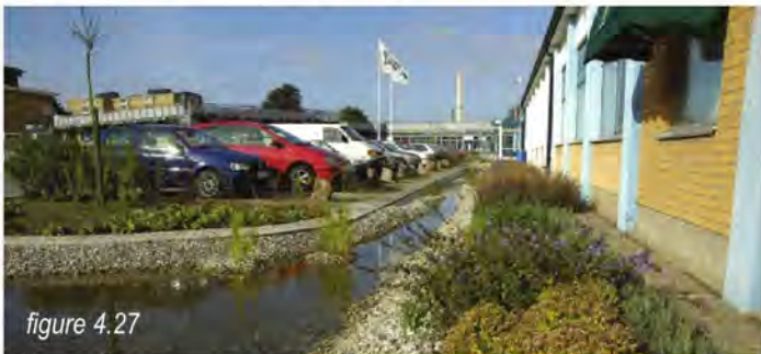
SWM should be integrated into Employment Areas and designed to be complementary to surrounding development.
