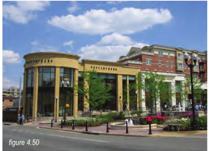
Buildings that occupy corner or gateway sites should include highly articulated façades.
