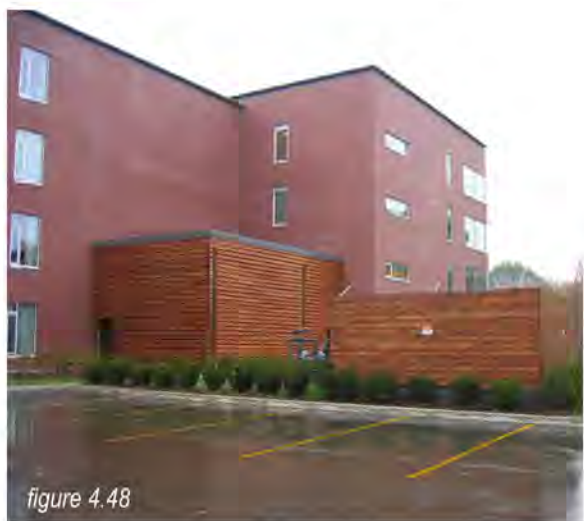
The design of service and loading areas should be integrated into the overall building and site design and feature durable materials of high quality and aesthetic value.
