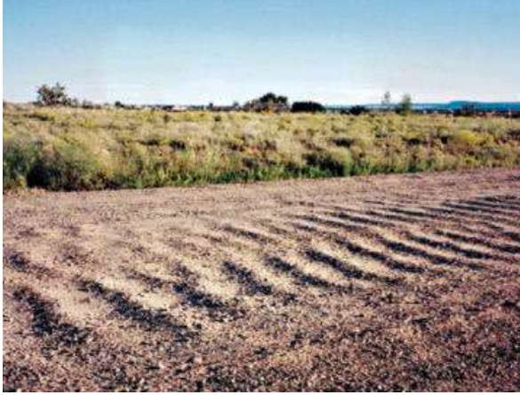
Figure 21: Washboarding Example (Photo from King Not Available)
