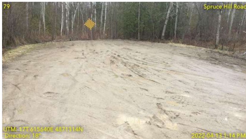
Figure 19: Spring Breakup Example
